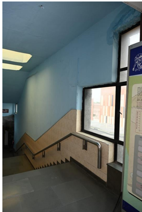
Fig 1.4 Gallery Entrance Right Wall
